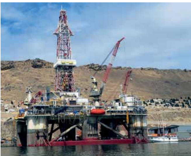
The Istiglal rig underwent upgrading and refurbishment at CSC with support from commissioning and production supervisors from Keppel FELS
